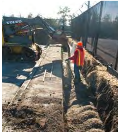
MTA Bus Depot Engineered Wetland
