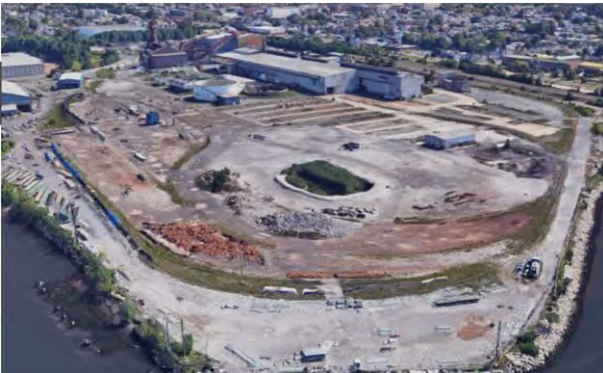
Distribution Ctr, Perth Amboy, NJ Clean Fill & Site Elevation
