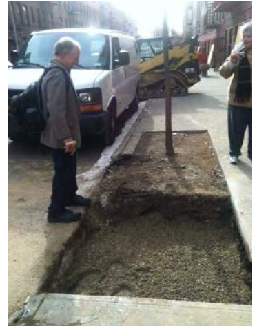
NYC Parks Department Stormwater Capture/Storage
