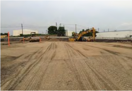
NJ Turnpike Interchange Sub-base & Embankments
