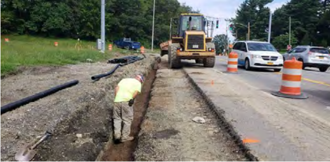
NYS DOT Yorktown lane widening project Underdrain Medium
