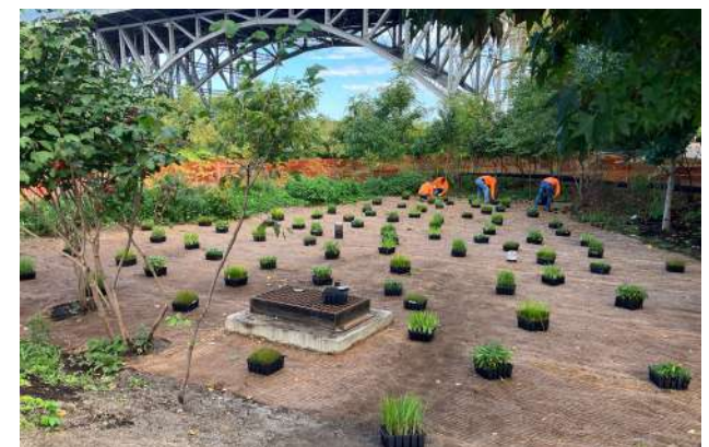
In partnership with Philadelphia Parks & Rec, the research team installed the soil blend in a Fairmont Park bioretention basin.
