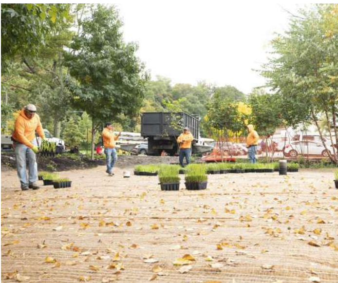
Figure 13: Installation of plant plugs.
