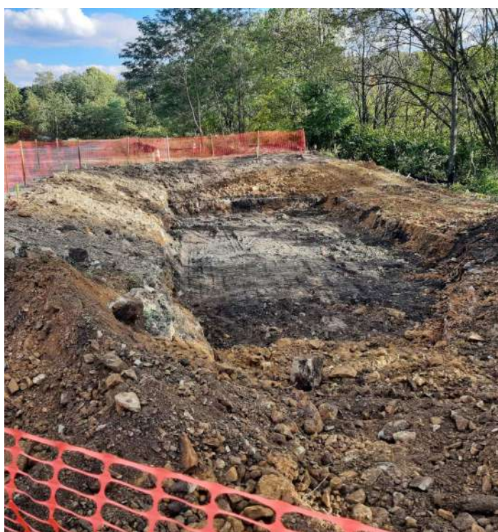
Figure 2: Rain garden under construction.
