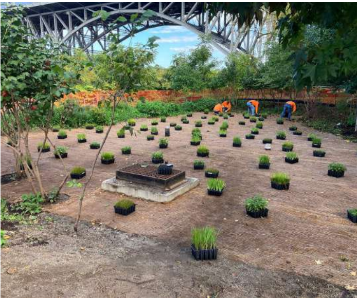
Figure 12: Laying out plugs prior to installation.
